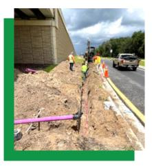
Work in preparation for landscaping began in 2023, including installing electrical lines, irrigation and water meters, as well as installing planting soil. FDOT and the landscaping contractor worked closely with Seminole County staff, as the county will be maintaining the landscaping. The contractor anticipated beginning plant installation in early 2024.
