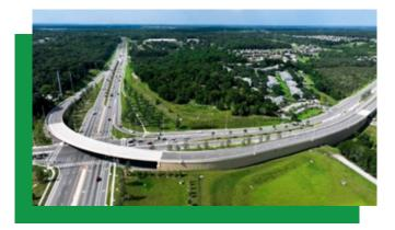
The project included converting the former U.S. 441 / S.R. 46 interchange into a more modern, signalized intersection with a flyover bridge. Work included installing medians, streetlights and pedestrian and cycling improvements. The opening of the flyover bridge in September 2020 represented one of many safety and mobility milestones for this project in Lake County.
